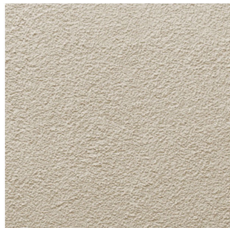
12. EXISTING RENDERED CONCRETE
