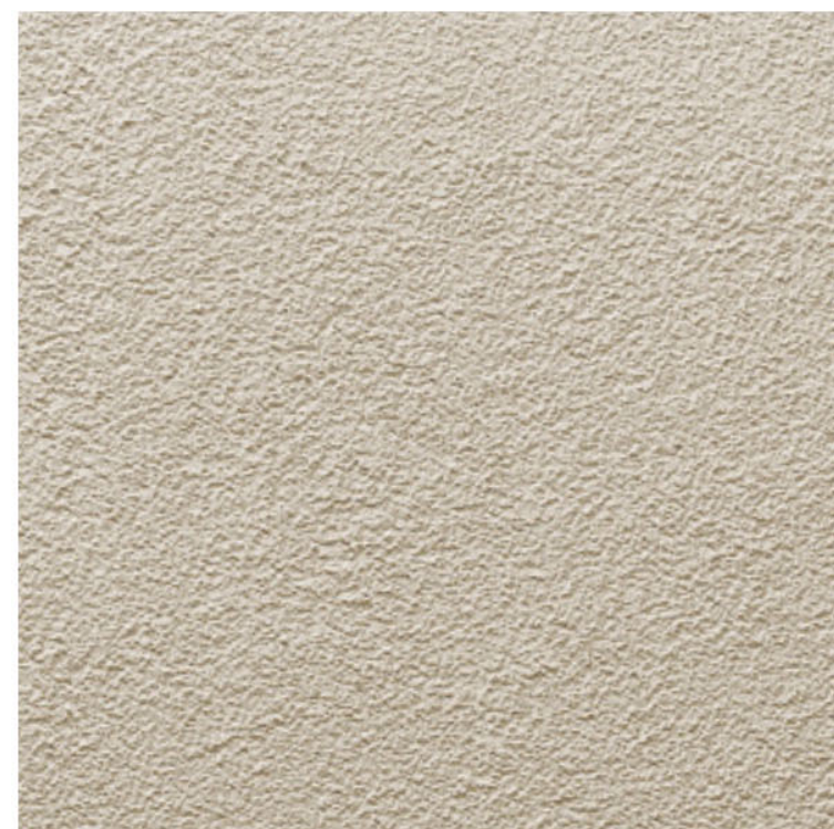
12. EXISTING RENDERED CONCRETE
