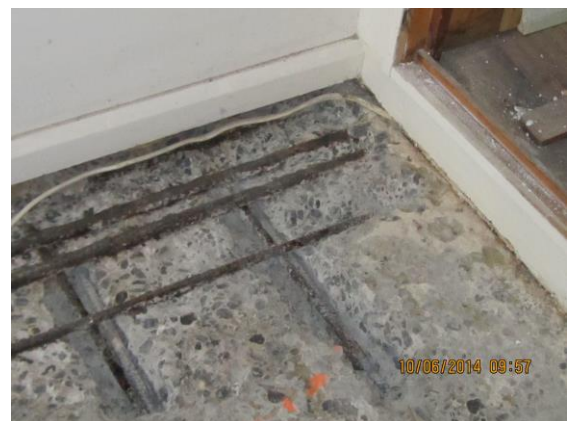
Photo 2: Close up of rebars that will be replaced.
