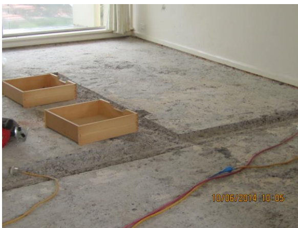
Photo 1: Unit floor stripped of magnesite .
